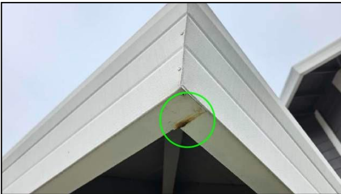
38. Evidence of gutter leak
