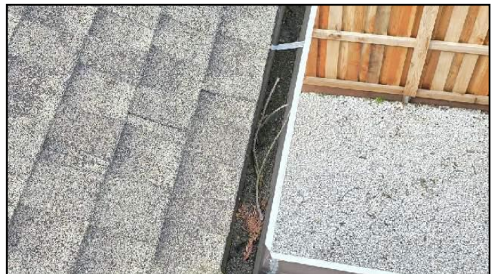
41. Debris in gutter
