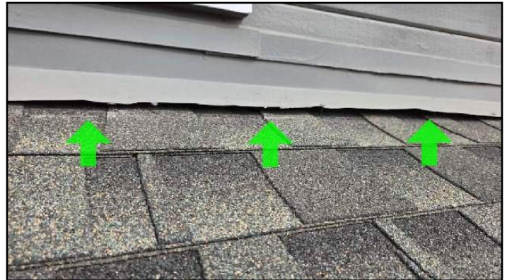
18. Lifted roof to wall flashing detail
