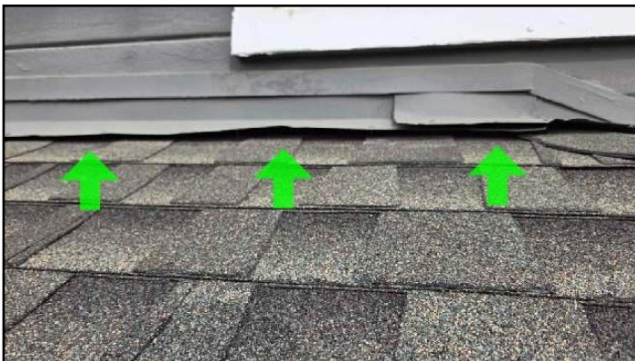
15. Lifted roof to wall flashing detail
