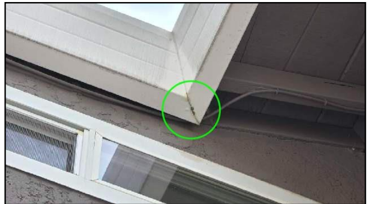
39. Evidence of gutter leak
