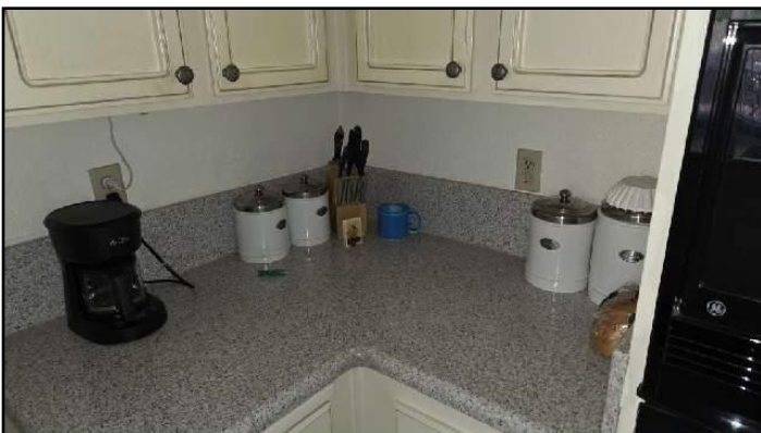
73. Outlets not GFCI protected
