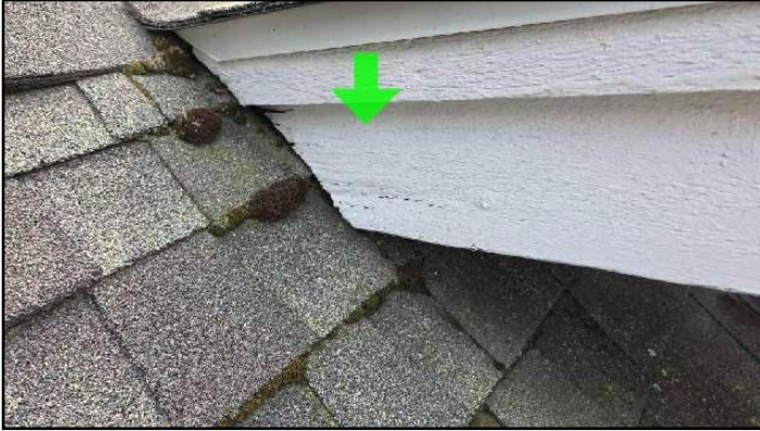
43. Upper level side yard eave
